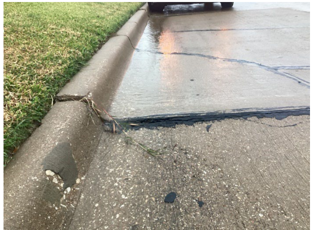
Displaced concrete
