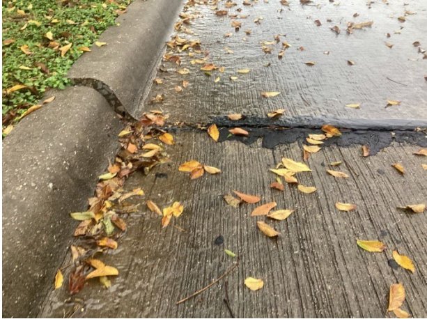
Displaced concrete
