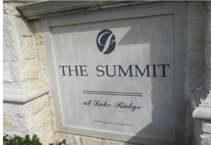
Cast stone signage is in very good condition.
