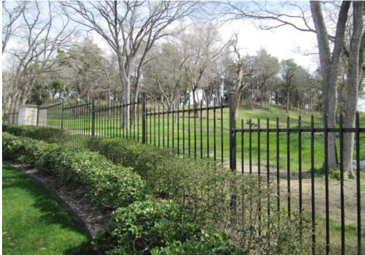
Overview of metal fencing at property entrance.
