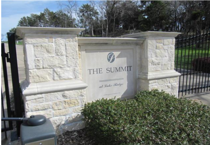
Cast stone signage at front property entrance.
