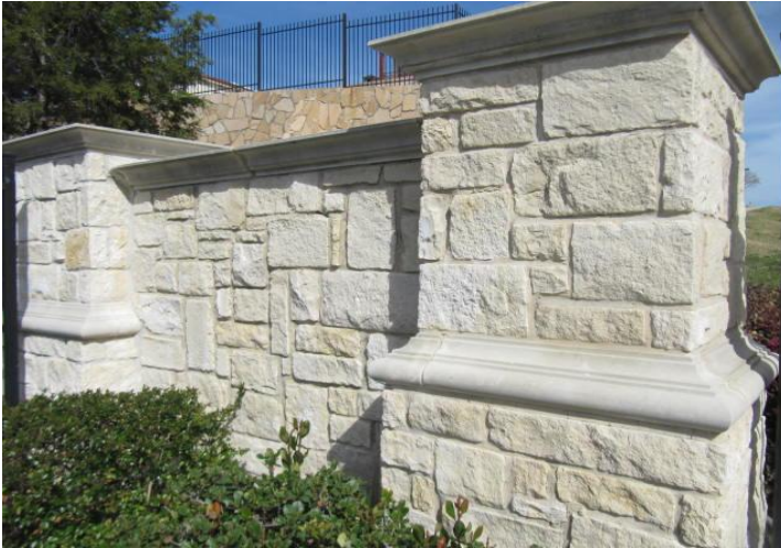
Rear view of masonry signage wall, at property entrance.
