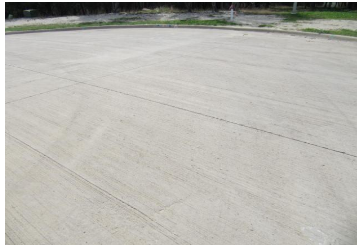
Typical surface condition at concrete street.
