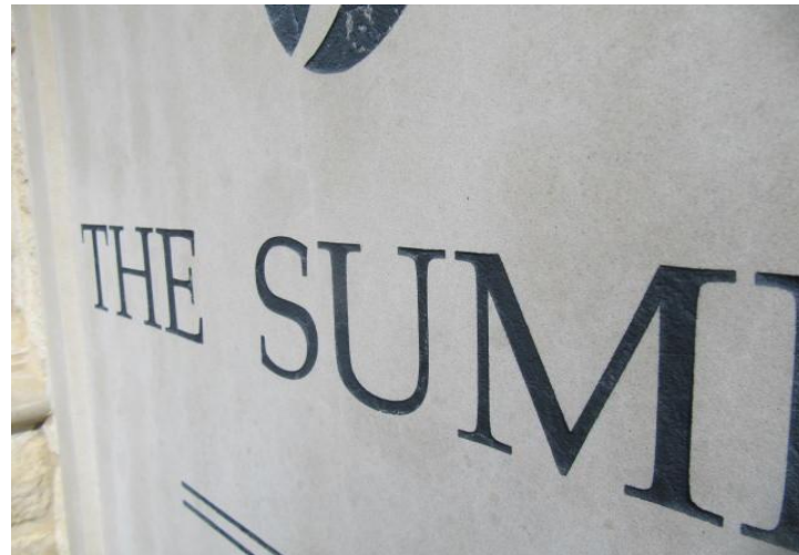
Etched lettering at cast signage.
