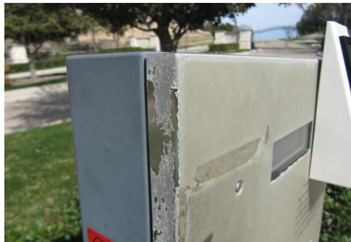
Worn finishes at side of intercom panel.
