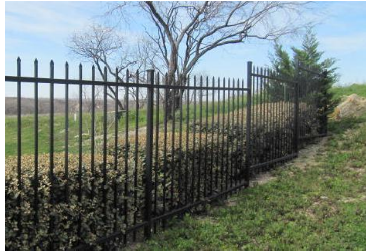
Typical style of metal picket fence.
