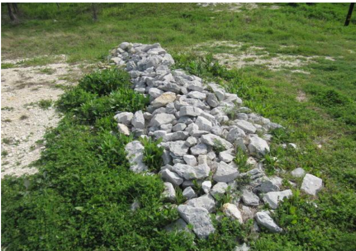
Typical condition of rip-rap at side of street.
