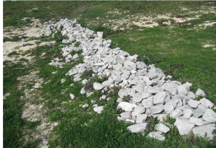
Rip-rap prevents erosion at steep hill.
