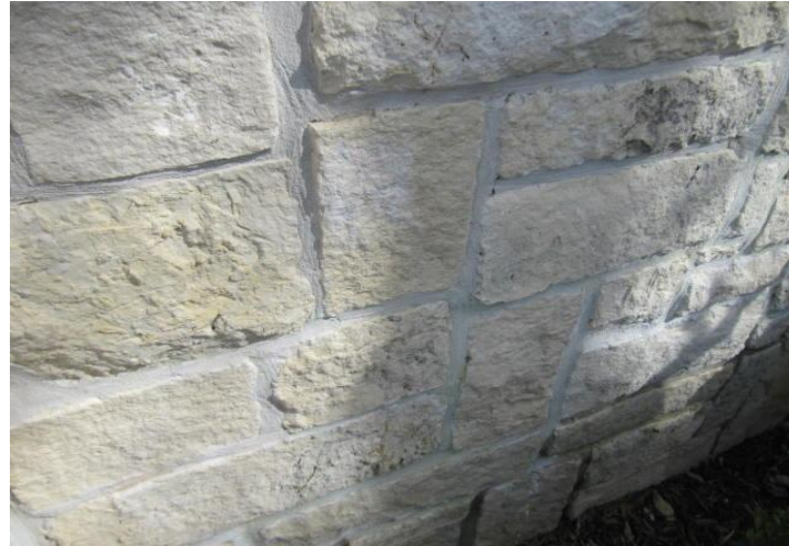
Masonry wall in good overall condition.
