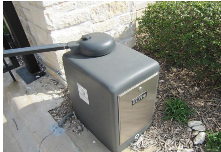
Typical swing gate operator.
