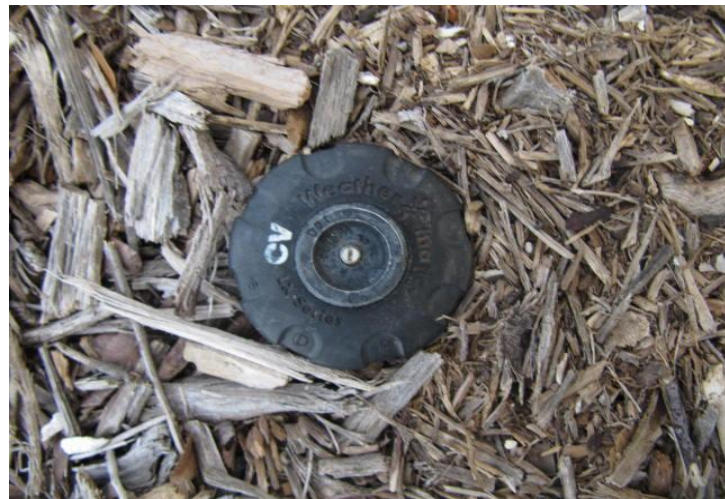
Typical irrigation sprinkler head.
