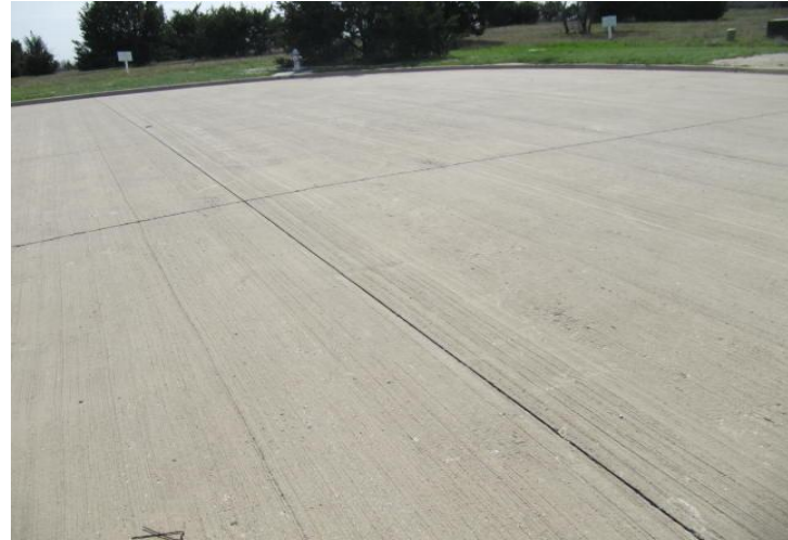
Streets are in good condition, with no visible cracks.
