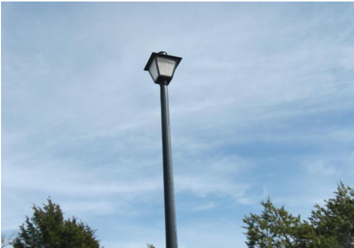
Light poles and fixtures are in good overall condition.
