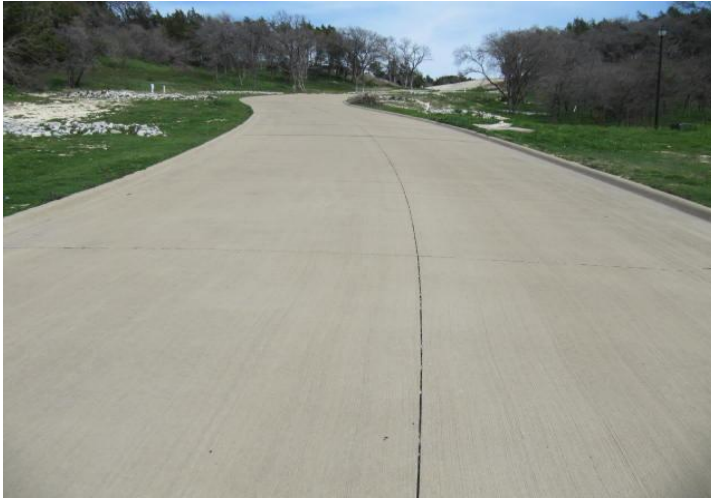
Overview of concrete street.
