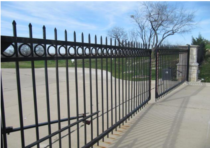
Swing style gates are in good overall condition.
