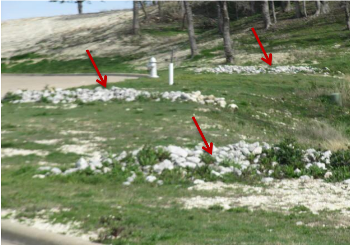
Overview of rip-rap at hill.
