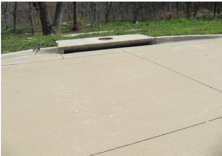
Concrete street, with raised curb and drop inlet.
