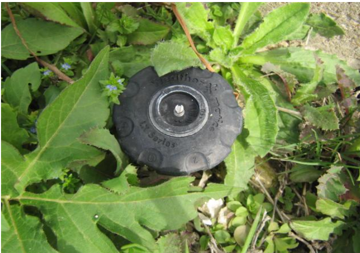
Typical irrigation sprinkler head.
