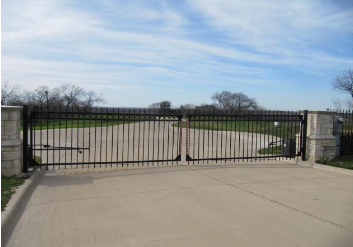
Overview of gate at rear property entrance.
