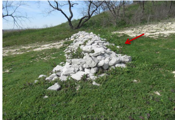
Higher grade at one side of check dam.
