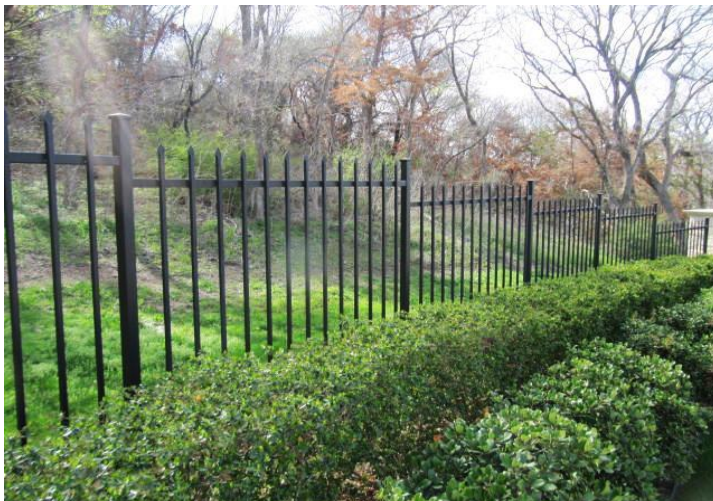
Metal fence near main property entrance.
