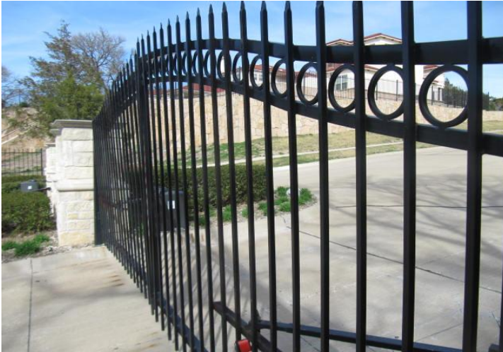
Overview of painted metal gate at property entrance.
