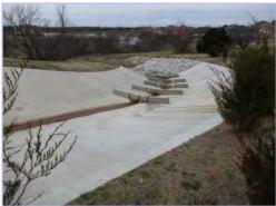
Drainage is a significant issue throughout the community. Drainage swales should be cleaned regularly and rip-rap replaced as needed. Areas should be inspected following each major weather event. Funding anticipates future projects to maintain the systems in proper working order.
