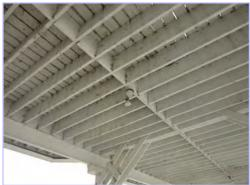
The deck substructure consists of metal and wood framing attached metal columns. The frame is showing signs of rust and deterioration in some areas. We anticipate an ongoing program of truss and post replacement to maintain deck integrity.
