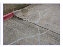
The concrete parking at the Ridge View Park and clubhouse area is in poor condition with areas of cracking and surface deterioration, but no pot holes or depressions. Surface integrity is critical to mitigate any subsurface moisture which will accelerate deterioration. Funding is to replace approximately 10% of the concrete on a regular basis.
