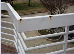
Metal fence and railing surface appears in overall fair to poor condition. Metal surfaces have a powder coated finish that once damaged will require restoring and protecting surface from moisture. Due to prohibitive costs of removing metal to re-powder coat, funding anticipates regular cycles of paint, utilizing a high quality exterior metal surface product. Remove rust and apply a rust inhibitor prior to painting.
