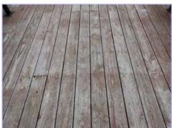
The wood decking surface sealer located at the community center appears in overall fair to poor condition with noted areas of fading or missing sealer. Recommend periodic inspections to ensure proper maintenance, repair any damage, and verify if deterioration is consistent with expectations. Seal regularly to prevent moisture penetration which will accelerate deterioration.
