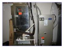
The gas furnaces are located in the rental floor area and appear to be in overall good condition with install dates ranging from 2000 to 2016. Recommend regular service in accordance with manufacturer's guidelines to ensure full useful life. Funding anticipates continued replacement of units an an as needed basis with no anticipation of replacing all units at one time.
