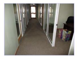
The rental area hallway and common area carpet, which includes the stairs and turret, is a typical medium grade commercial carpet and is in worn and stained condition in areas. Recommend regular cleaning to maximize useful life.
