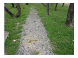
The gravel walking trail at Fossil Ridge Park is in overall fair to poor condition with extensive areas of cracking. Recommend repairing any trip/fall hazards immediately and inspect regularly for any damage. Funding is to repair sections as needed, with no anticipation of replacing all of the trail at one time.
