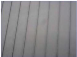
The corrugated metal roof on the clubhouse appears in overall good condition and is reported to have been replaced in 2017. Recommend yearly inspections by a qualified roofer to ensure proper maintenance, repair any damage, and verify if deterioration is consistent with expectations.
