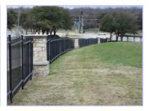
Metal is in fair condition with limited signs of rust or damage, but some broken welds. Fence has a powder coated finish that once damaged will require restoring and protecting surface from moisture. Due to prohibitive costs of removing fence to re-powder coat, funding is based on maintaining fence by treating rust and painting. Recommend periodic inspections to identify and treat damaged areas in order to avoid additional future costs to repair.
