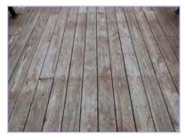
The wooden deck surface located at the upper deck (1,648 GSF), lower deck (1,075 GSF) and walkway (176 GSF), located at the community center is in overall fair condition with noted weathering of the wood sealer. Recommend repairing any trip/fall hazards immediately as noticed and inspect regularly for any damage. Reseal regularly to mitigate any subsurface moisture which will accelerate deterioration. Funding is to replace all decking at one time to maintain consistency and appearance.
