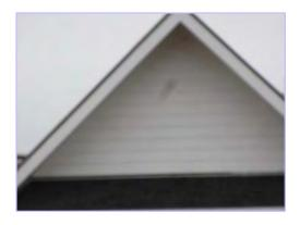
Paint is in generally good condition with minimal areas showing signs of fading, peeling, dry and missing or cracked caulking. Recommend caulking around areas of wood to brick transition. Preventing moisture penetration via cracks (wood shrinking around transitions) is key in ensuring a full useful life.
