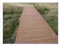
The wood bridges at the Ridge View Park walking trail appear in overall fair condition with slight fading and damage to the wood surface noted. Recommend regular staining or painting to protect wood, and periodic inspection to secure loose components. Anticipate eventual replacement of the wood deck and some structural components due to use and exposure to the elements.
