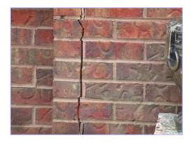
The brick veneer siding appears in overall good condition with no noted areas of damage or missing grout, but one small area of cracked brick, possibly from foundation movement. Recommend periodic inspections to ensure proper maintenance, repair any damage, and verify if deterioration is consistent with expectations. Repoint brick periodically to prevent subsurface moisture penetration which will accelerate the deterioration of this component.
